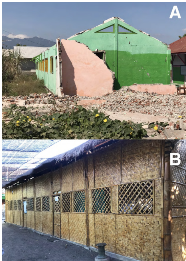
Figure 13 Photographs of (A) a school destroyed by the 2018 Lombok earthquake series, and (B) a bamboo school built after the earthquakes. Teachers struggled to get students to attend school in the new building due to its construction style.
