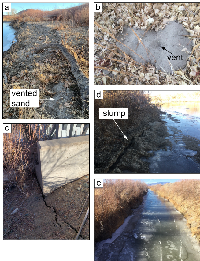
Figure 6 Field photos of secondary shaking effects. (a) Zone of lateral spreading along the bank of the Walker River. Pockets of sand ejecta (bottom right) bury leaf litter (39.1560, -119.0863). (b) Liquefaction-related sand boil along bank of Walker River. Collapsed vent is in the center of the deposit. Sand cleared away on left to demonstrate leaf litter buried by the sand (39.1571, -119.0864). (c) Power line road bridge over the Walker River. Cracking and separation (up to 3 cm) of fill from south concrete abutment. (39.1587, -119.0515). (d) Riverbank slump in terrace deposits below south abutment of power line road bridge (39.1585, -119.0517). (e) Cracked and healed ice in frozen drainage ditch (39.1514, -119.1042).
