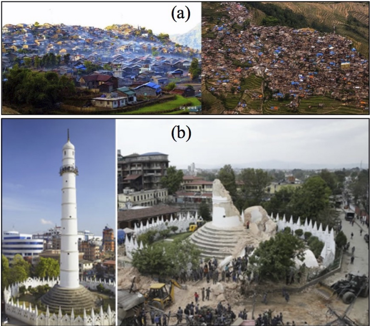
Figure 1 Examples of damage from the 2015 Gorkha earthquake. (a) Gorkha Barpak (epicenter village) before and after the Gorkha earthquake when the earthquake destroyed almost all houses (Adhikari, 2021). (b) Historic Kathmandu tower “Dharahara” before and after the 2015 Gorkha earthquake (Shrestha, 2016).
